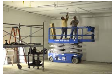
Archive of Visual Arts Building (AVA) During renovation July, 2011
